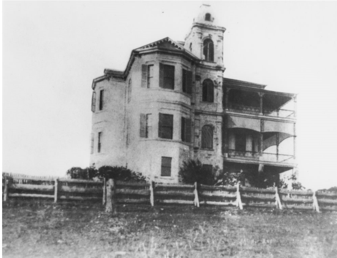
Image 5: San Souci, later Palma Rosa, designed by Stombuco in 1886 as his own home. Note the central arch-windowed turret and triangular pediment, and the way the structure extends out in octagonal sections to the left. Source: State Library of Queensland.
