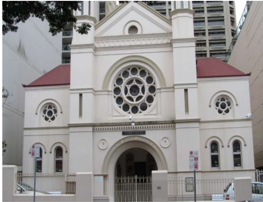
Image 1b : The Brisbane Synagogue, photographed in the 2000s. Note the two flanking turrets and upper triangular pediment with window, the large central rose stained glass and smaller horseshoe-shaped windows, and the dentils and decorations in the stucco on the outer face of the synagogue. Source: State Library of Queensland (a), Brisbane Hebrew Congregation (b)
